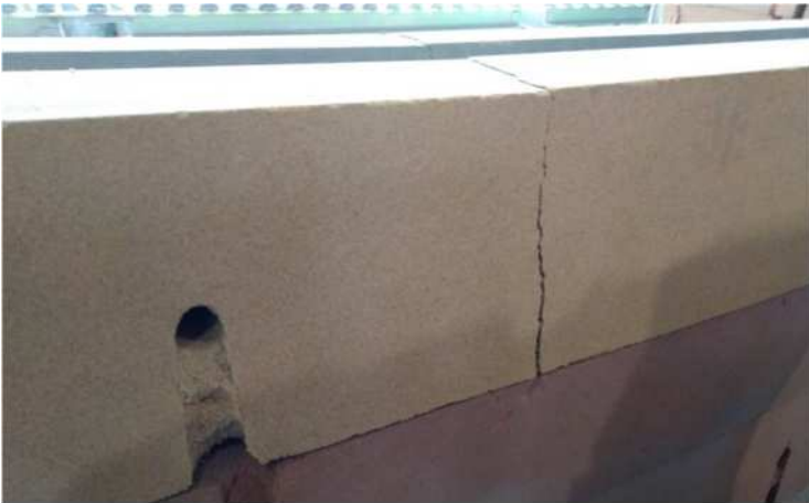
Figure 14. Mould made by Geopol, broken after stripping.
