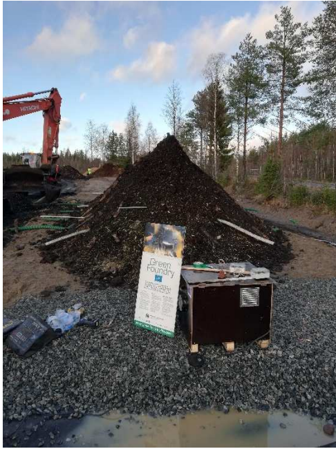
Figure 27. Test heaps under construction.
