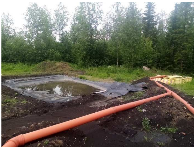
Figure 21. Wastewater collection system
