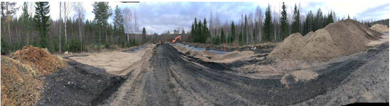
Fig. 4-5. Constructing the composting test field.
