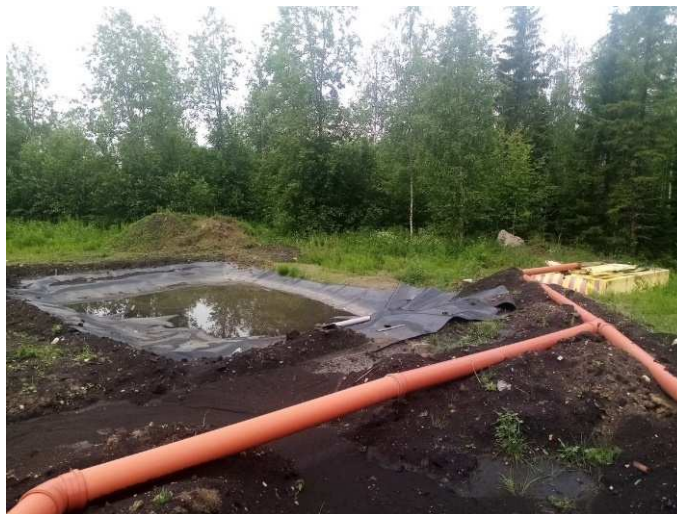
Figure 21. Wastewater collection system
