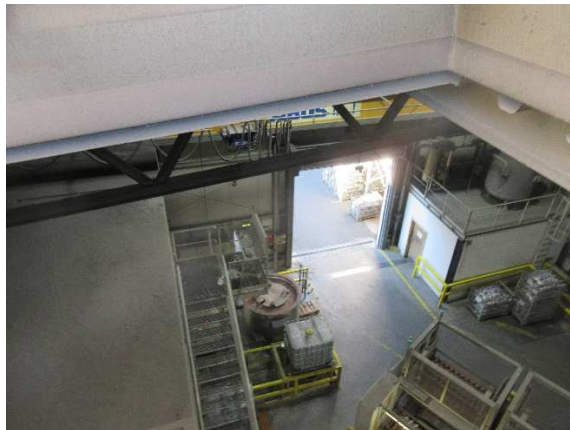
Picture 2. Open outer door
