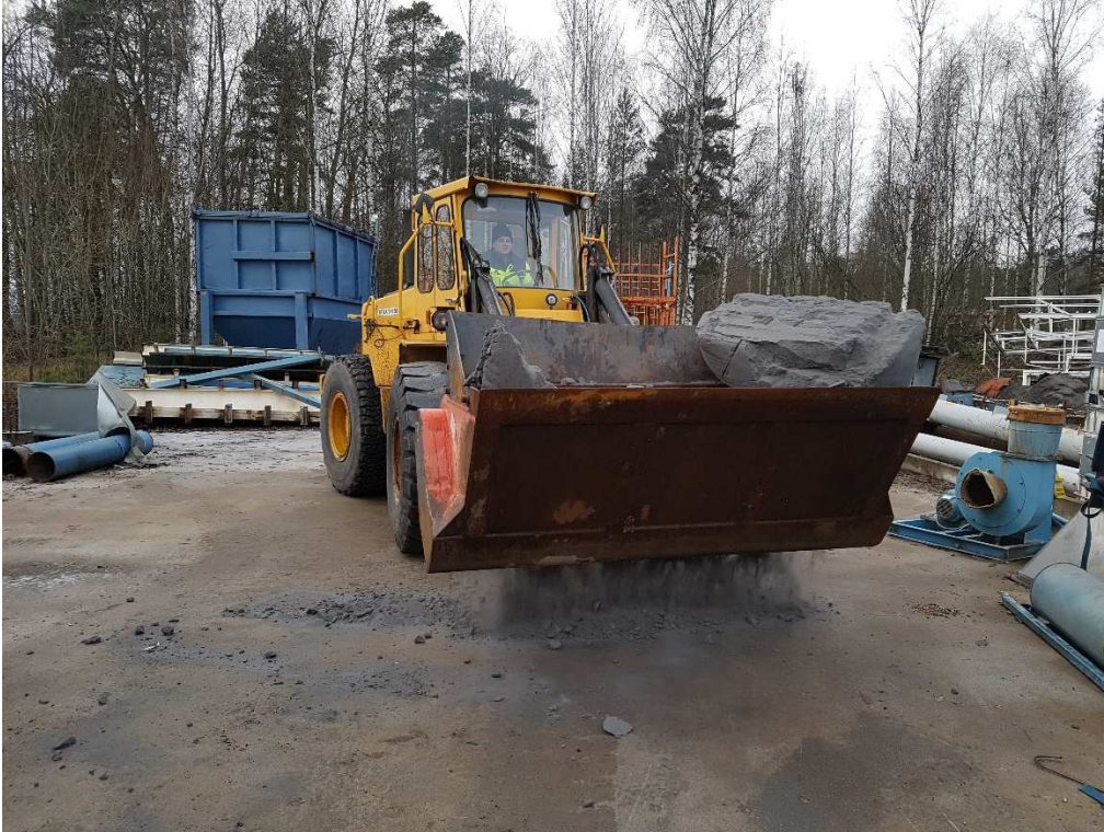
Fig. 2 Crushing Inotec sand with a bucket crusher
