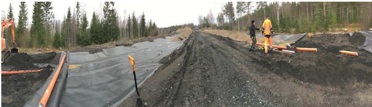
*Figure 5: Setting up a composting plant. A watertight film was installed and waste water collected from the site in a separate water tank.*
