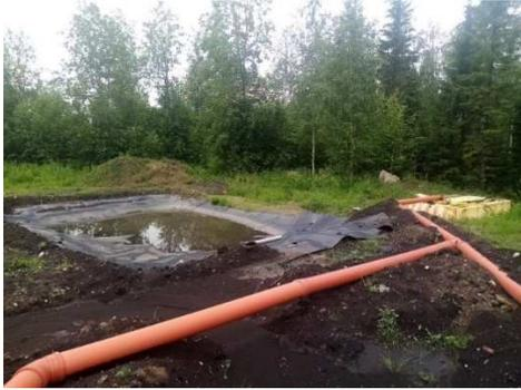
Fig. 19. Wastewater collection pipelines, a container and overflow basin.
